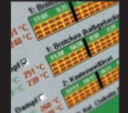
The user-friendly control system guarantees optimum baking processes that can be reproduced whenever required
